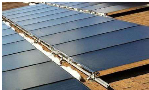
Fig.12. Flat Plate Collector [32]
