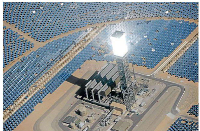
Fig.9. Ivanpah Solar Power Plant [25]
