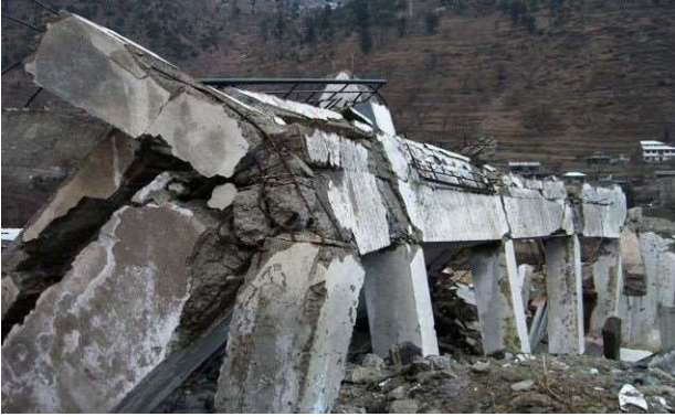
Fig. 2. Failure of beam column joint in Kashmir earthquake 2005
