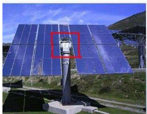
Fig. 4. High precision solar tracking drive [20]
