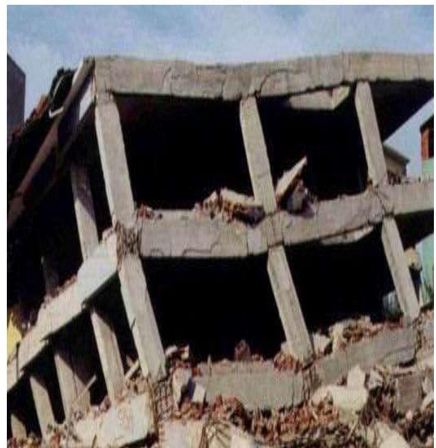
Fig. 1. Structural collapse during 1999 Kocaeli earthquake, [2]
